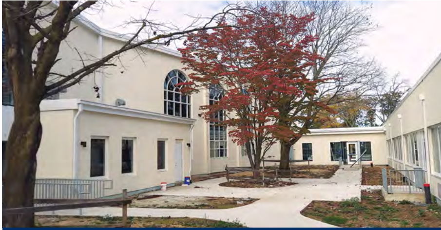
COURTYARD GARDENS WORK IN PROGRESS
