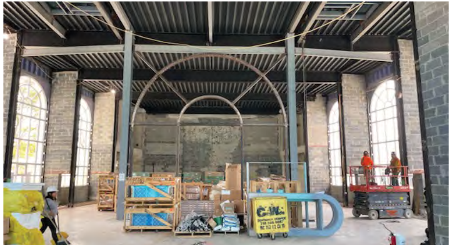
MAIN LOBBY AND VIEW OF FUTURE CHAPEL
