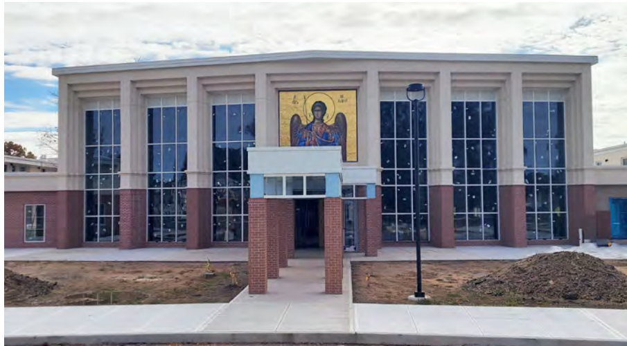
FINAL WORK ON THE ENTRANCE AND FACADE
