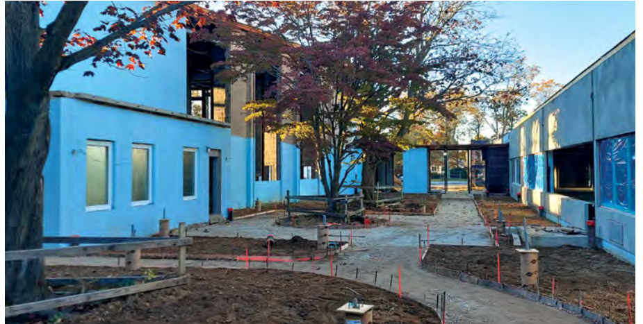
COURTYARD GARDENS WORK IN PROGRESS
