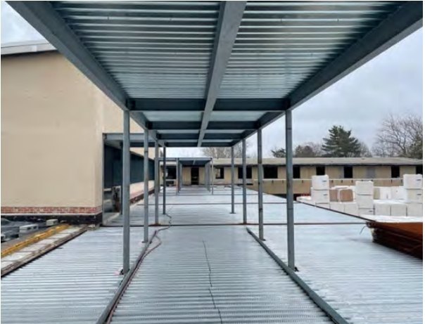
ERECTED STEEL AND DECKING FOR MEMORY CARE WING
