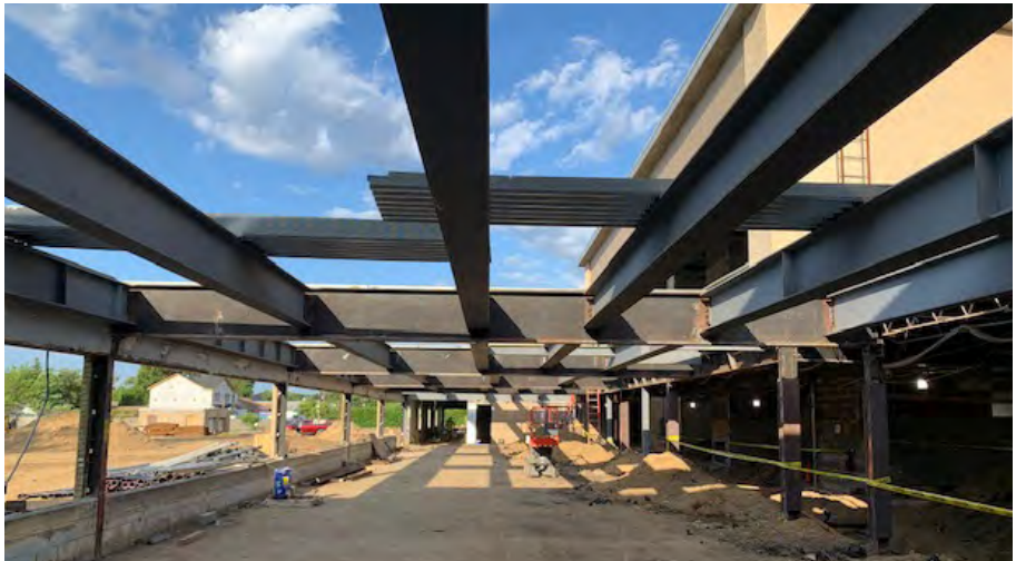
ERECTED STRUCTURAL STEEL FOR WING CONNECTOR
