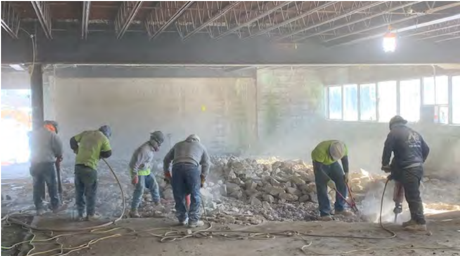
SLAB ON GRADE SECTION BEING DEMOLISHED
