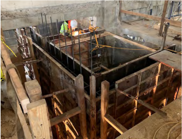
ELEVATOR SHAFT READY TO BE POURED
