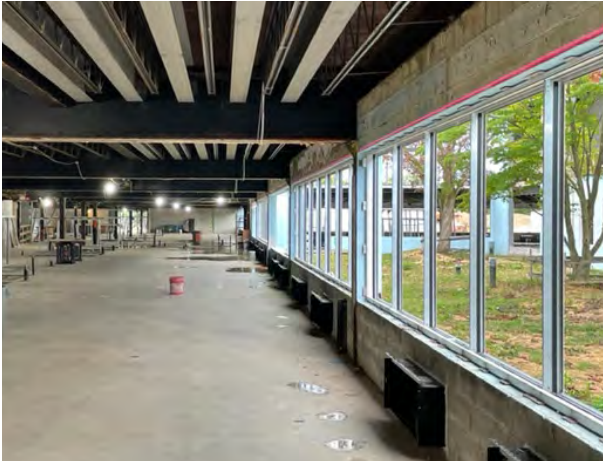
INSTALLED WINDOW FRAMES IN EAST WING
