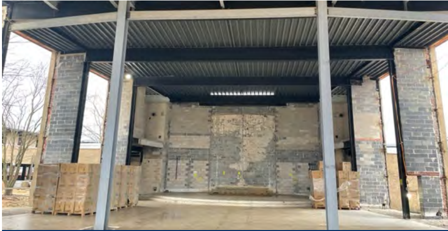
NEW CHAPEL INTERIOR FACING FUTURE ALTAR AREA
